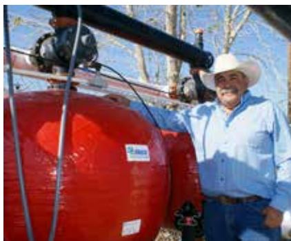
THE FIVE-FILTER STATION CAN BE EXPANDED WITH ANOTHER FIVE FILTERS AS NUNES INCREASES HIS ALMOND ACREAGE UNDER DRIP.
