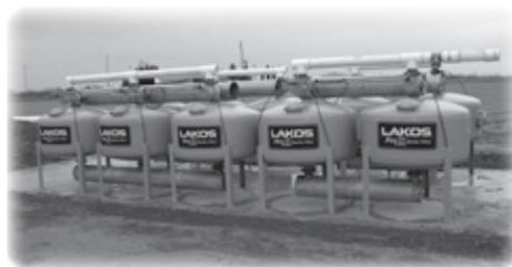
THIS NEWLY INSTALLED 10-FILTER SAND MEDIA FILTRATION STATION WILL SERVE SEVERAL DEL MAR OWNED OR LEASED FIELDS IN CCID UNDER DRIP IRRIGATION.
