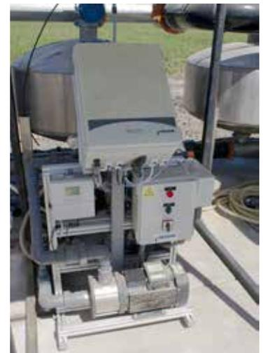
THE DRIP INSTALLATIONS AT LEWIS MAIORINO RANCHES ARE CONTROLLED BY FULLY AUTOMATED COMPUTER SYSTEMS THAT ALLOW IRRIGATION MANAGERS TO REMOTELY ADJUST PUMPS, FERTILIZER RATES AND IRRIGATION SETS, WHILE KEEPING RECORD OF HOW MUCH WATER AND FERTILIZER IS APPLIED AND WHEN.
