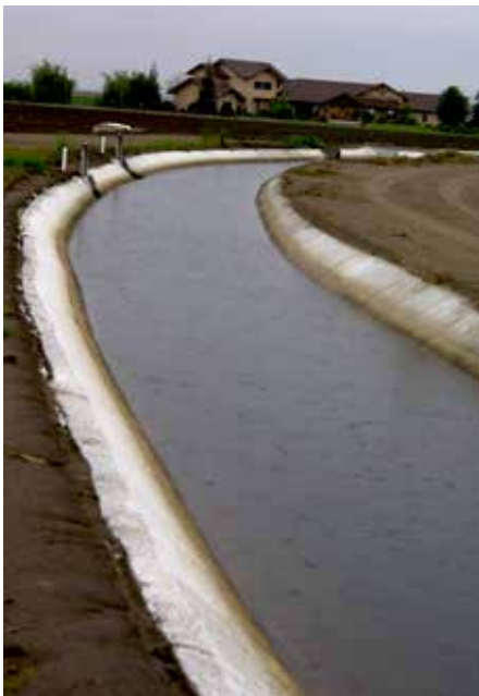
THE PROJECT ALSO STRAIGHTENED SEVERAL MEANDERING SEGMENTS OF THE DITCH TO IMPROVE DELIVERY TIME TO THE FARM.
